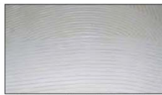
Example of properly troweled adhesive application
